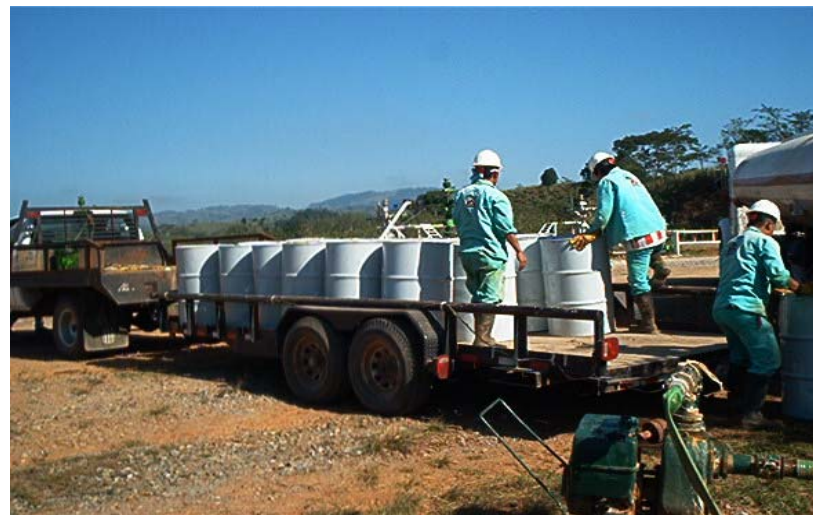
Fig. 2 Diluting SuperAll#38 in tank truck with water (1:8)
